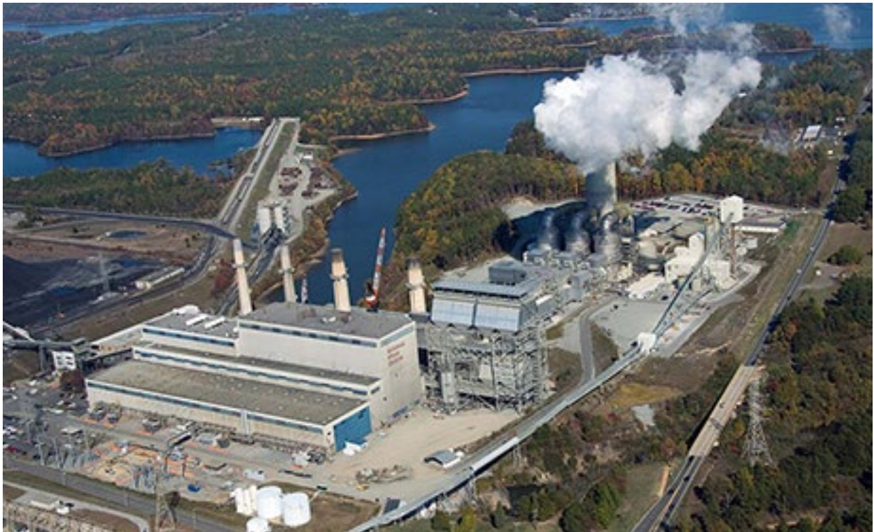
Marshall Steam Station Photograph
